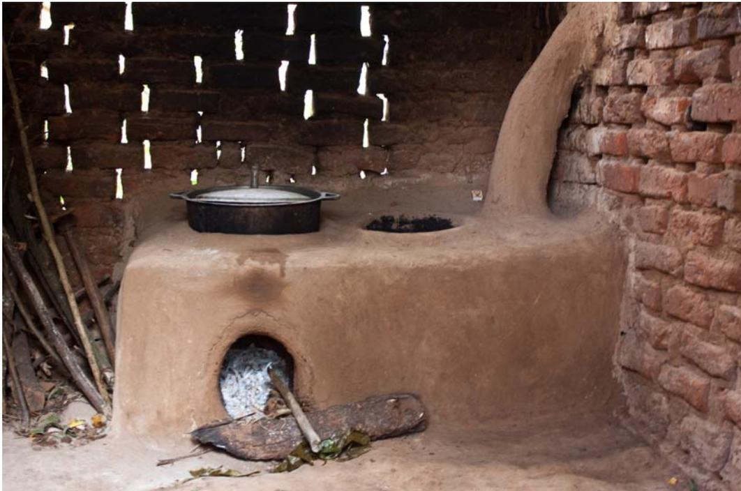
Figure 5.6b. Food is cooked on an energy efficient stove in Uganda, with smoke led out of the kitchen. It is fuelled by branches collected on the farm. (Photo: Vi-skogen, Ylva Johansson)
